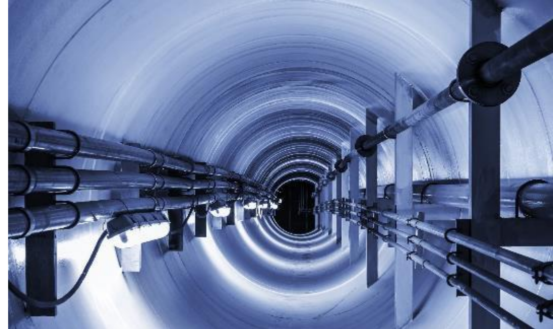
Diesel power plants Spain
