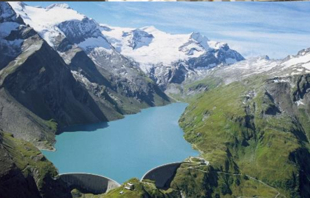
Kaprun Limberg II Hydro power plant Austria
